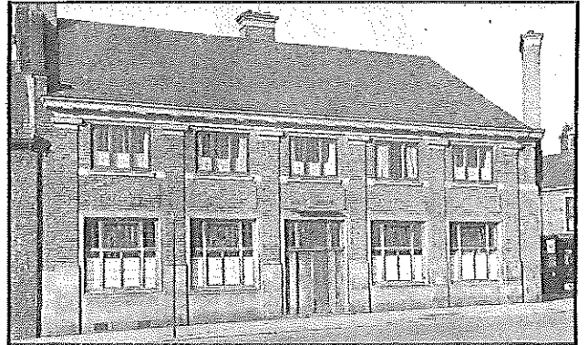
Malt Shovel after rebuilding
